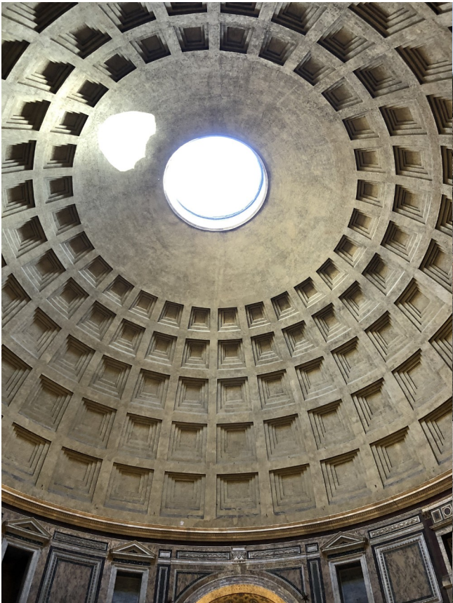
After two thousand years, the dome of the Pantheon is still the largest unreinforced concrete structure anywhere.
